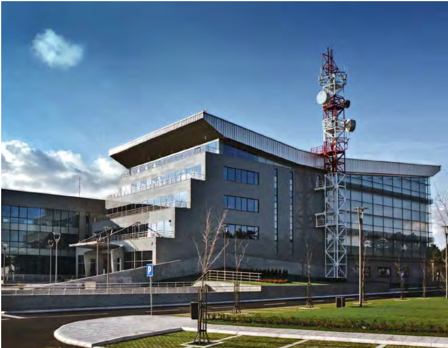
Figure 9: New ATC Centre Building
