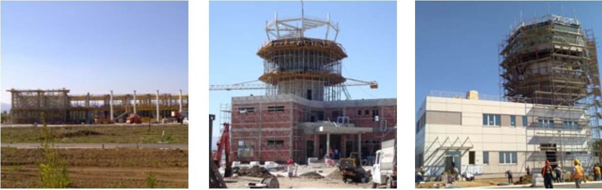
Figure 24: The construction of new ADC Kraljevo building
